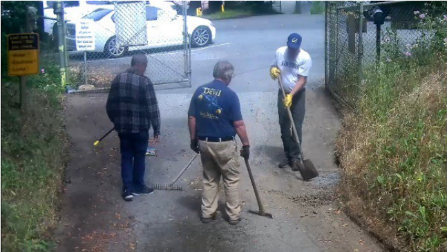
Bruce and Andy clearing the drain
